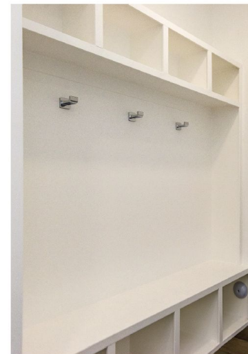
SITE BUILT MILLWORK FOR MUDROOM
