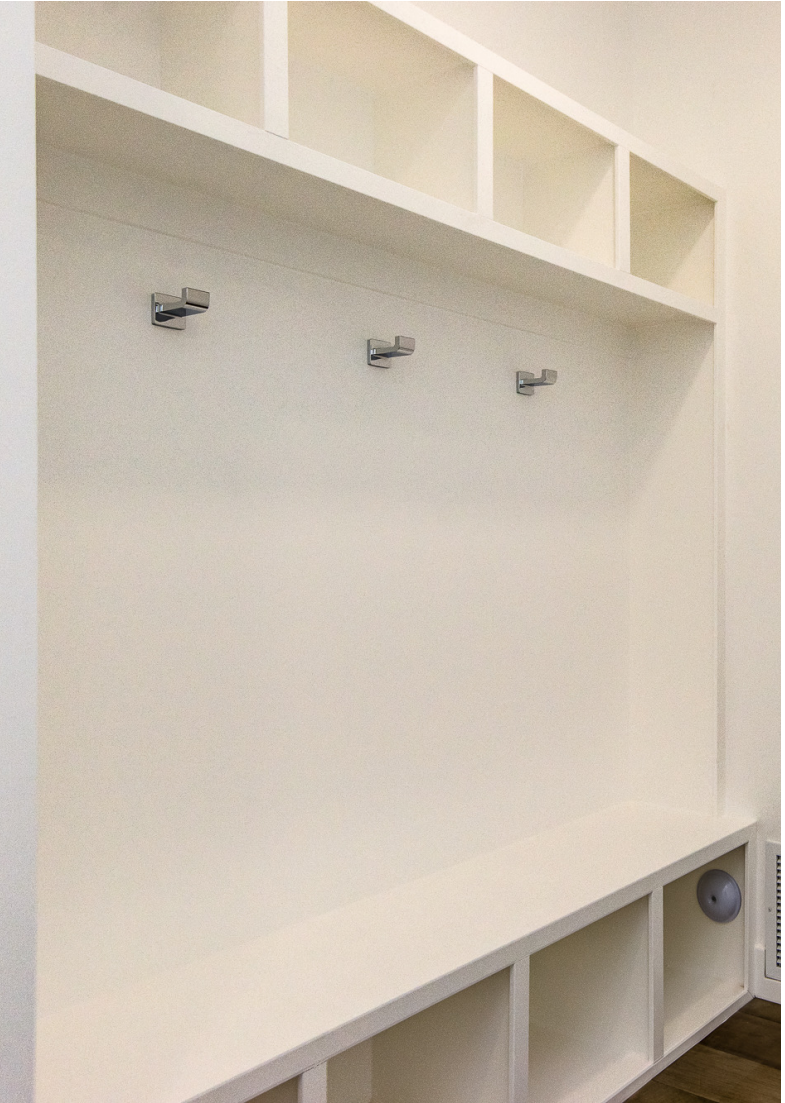
SITE BUILT MILLWORK IN MUDROOM
