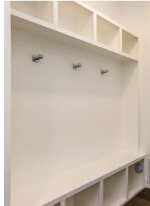
SITE BUILT MUDROOM
