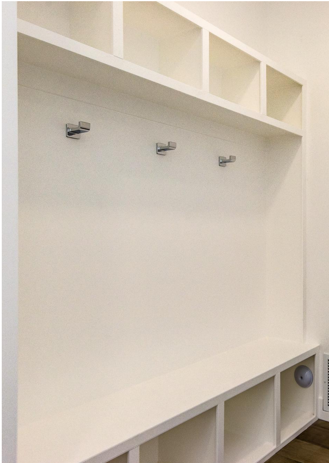
SITE BUILT MILLWORK IN MUDROOM
